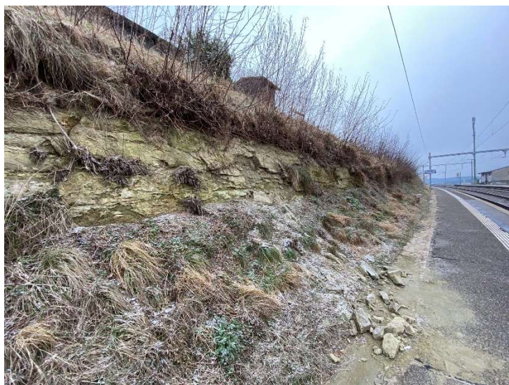
View of the eroded sandstone slope, prior to stabilization works
